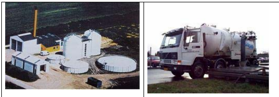
Figure 9.13 Filskov Centralised Biogas Plant (NNR, No date)
