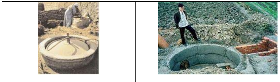
Figure 9.4 Small Scale Digester, India, (Wikipedia, 2006)
