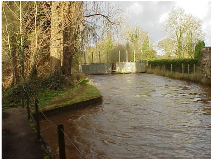
Figure 8.8 Headrace for run of the river hydro project (Tipperary Institute)
