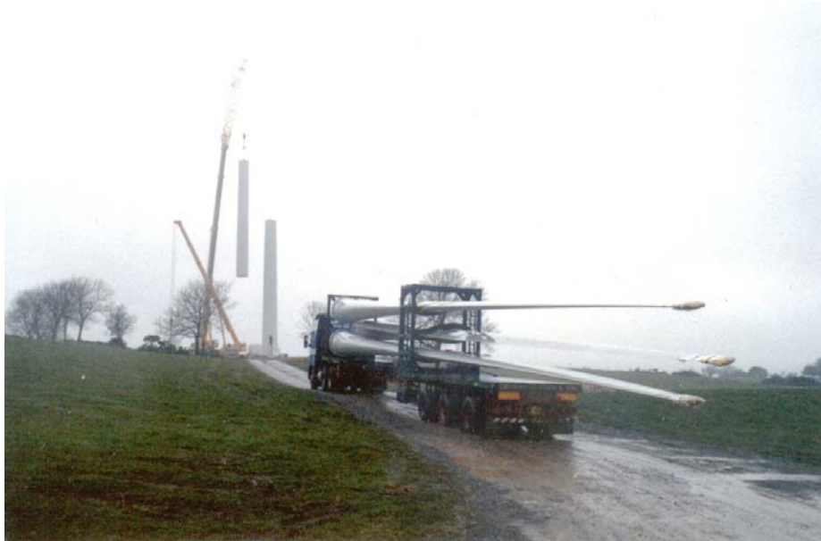
Figure 7.6 Blade delivery and tower construction (Tipperary Institute, 2005)
