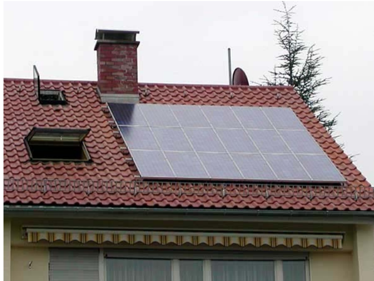
Figure 5.1 Roof Mounted Photovoltaics (Krannich Solartechnik; evergreensolar 2005)
