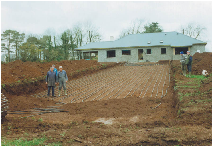
Figure 4.6 Horizontal collector installation at domestic dwelling (Dunstar, 2006)
